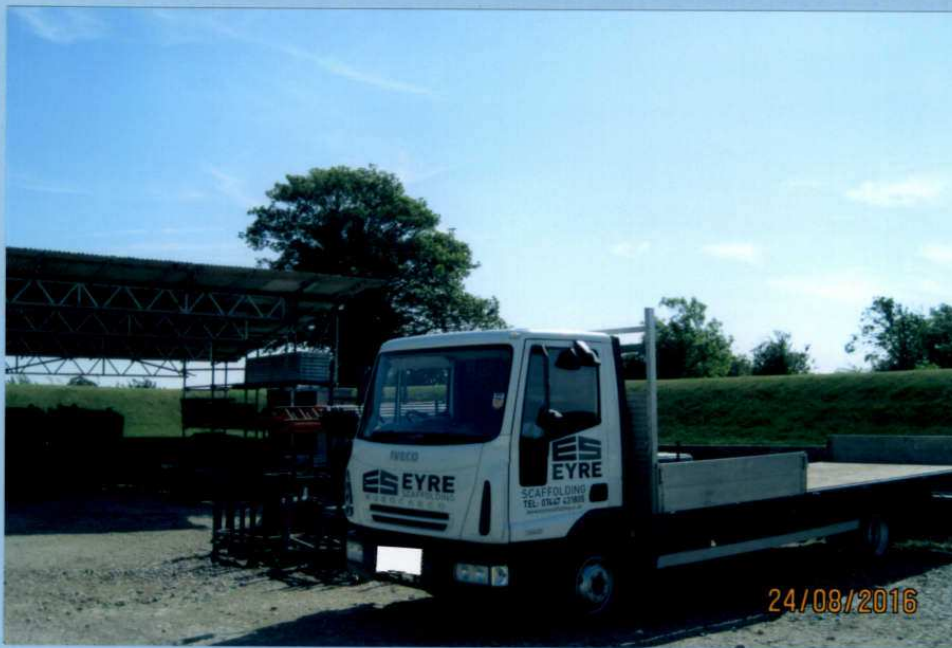
EYRE SCAFFOLDING. NOTE PROTECTIVE BONDING EMBANKMENT.
